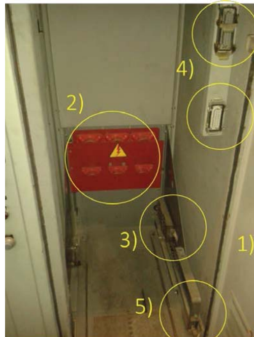
Figure 9. Original CB compartment renewal points
