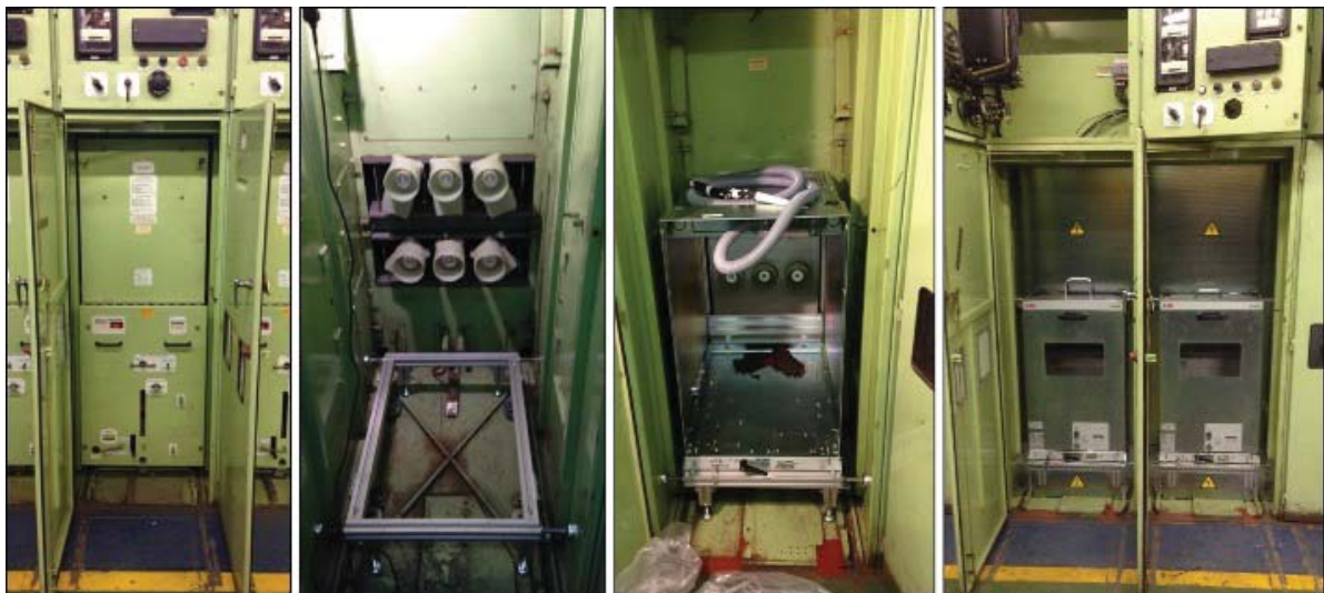
Fig. 5 Retrofill installation sequence
