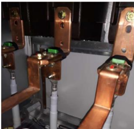
Fig. 13: Sensors installed on a cable connection of an MV cubicle with circuit breaker
