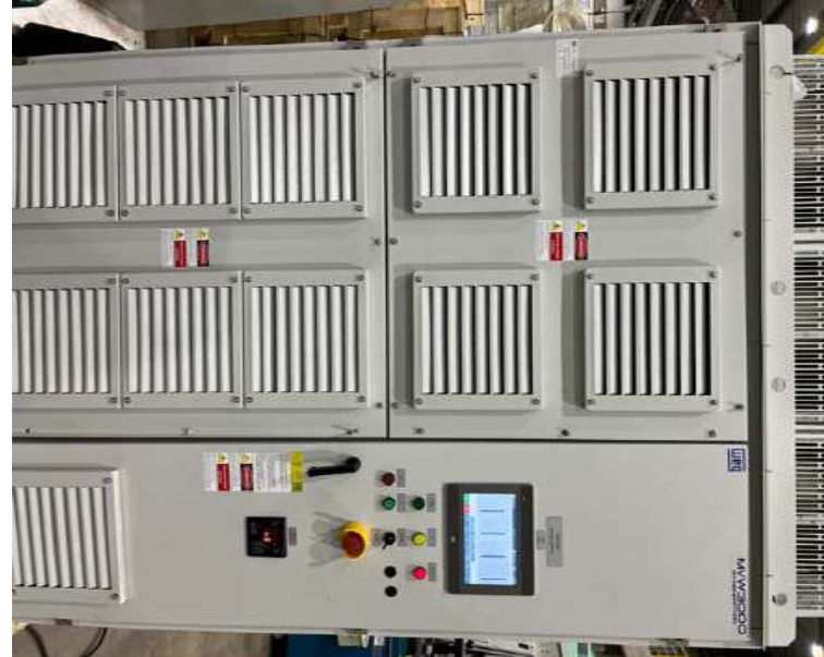
Fig 20. 70A/4160V Medium voltage Drive.
