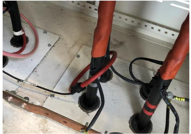
Fig. 21 Installation of Rogowski current sensors around MV cables.
