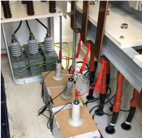
Fig. 20 Installation of capacitor voltage divider probes on customer site
