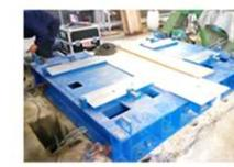
2. Key challenge → turbine separation from its tabletop foundations without damaging the concrete and skid installation
