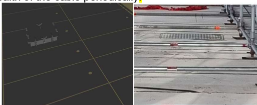
Figure 5 Cable Trench heat vent and inspection hatch
