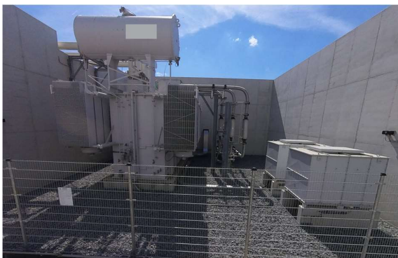
Figure 9 Main Intake transformer
