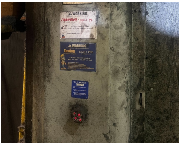
Figure 2 - Panel-Mounted PESD in Dirty Environment
