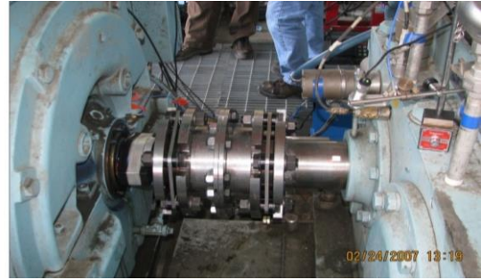
Figure 12. Installed Drive Train
